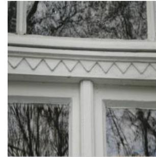
The design is according to test certificate driving rain-proof Class C. Hose seal in the sash available in white or brown.
